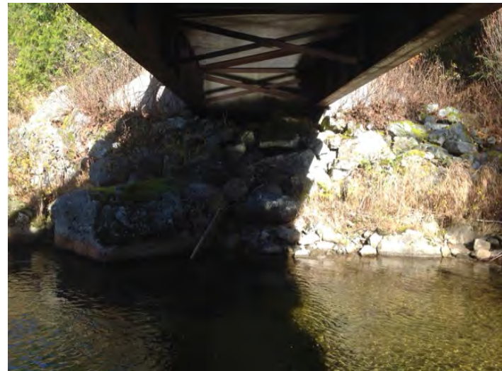
Left Bank Abutment when facing downstream
