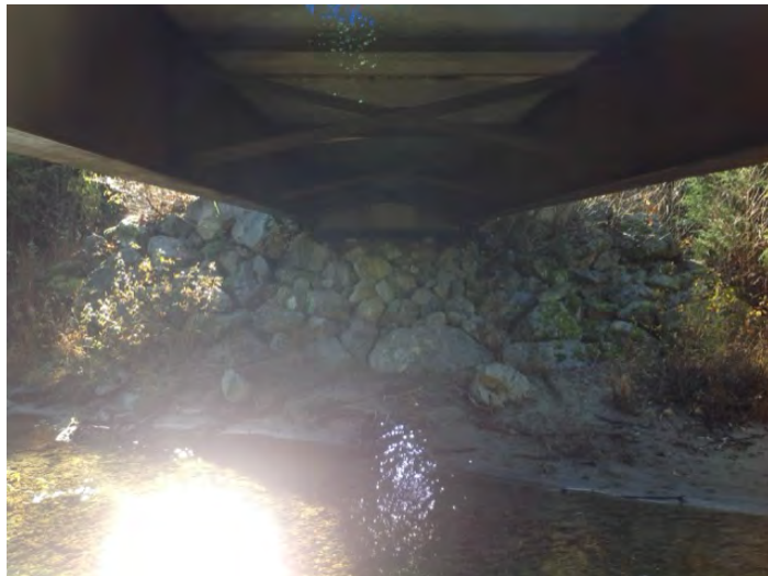
Right Bank Abutment when facing downstream
